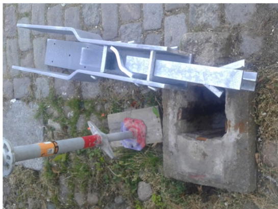
Fig. 6. Ny stolpsko innan montering.
